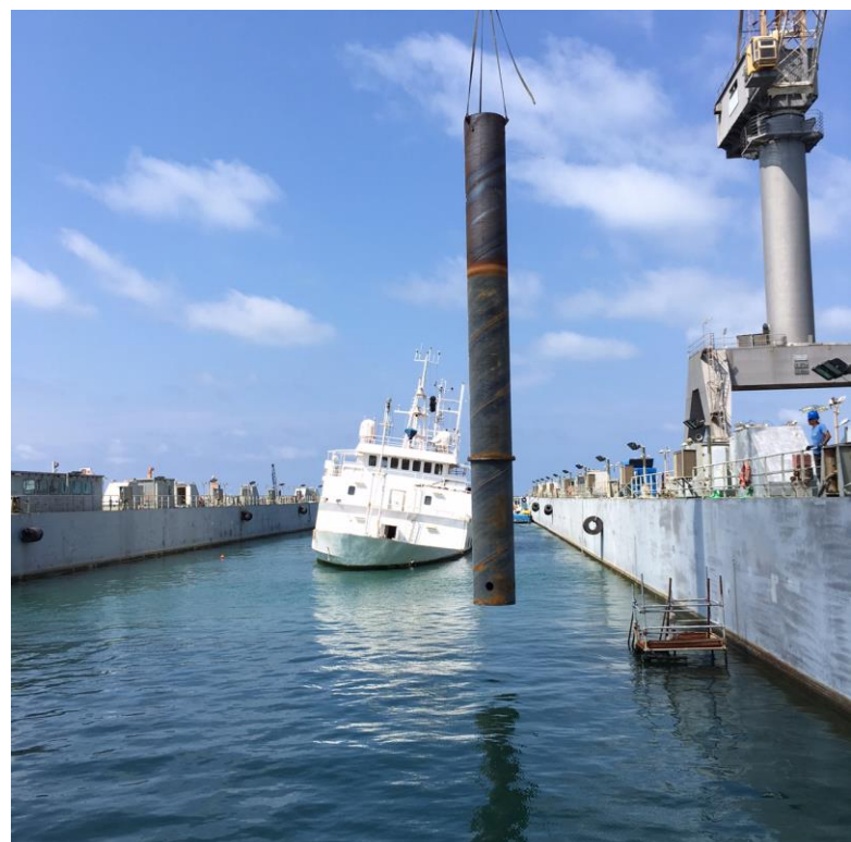
Figure 6. Lowering of pumping pipe into dock
