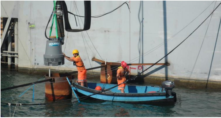
Figure 7. Lowering of pump into pumping pipe
